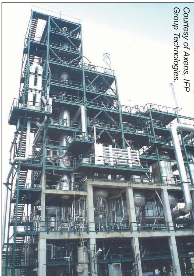
Figure 1. Continuous catalytic reformer (CCR).
