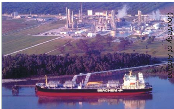
Figure 4. CosMar EB/SM facility, Carville, USA.
